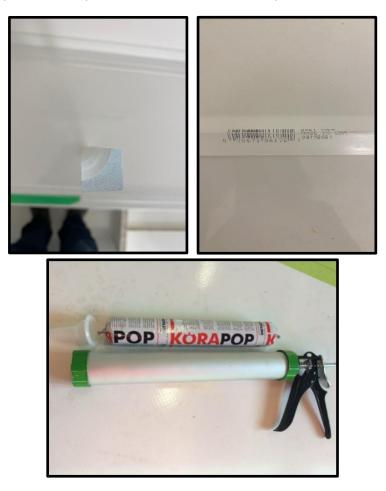
5. Glue should be applied on all edges and corners with the panel in place. We recommend using extra glue where the trim will be placed. Tape is also useful to secure the trim in place.
