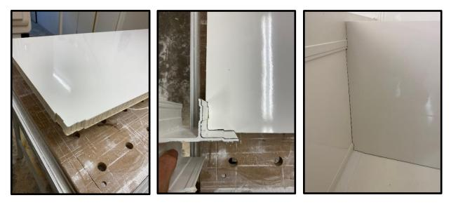
2. Before gluing panels in place make sure to clean areas with denatured alcohol and a clean rag.
