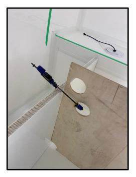
4. We recommend the use of Koemerling Korapop adhesive to secure the panels into place. We also recommend using PVC trim (available from Home Depot). The trim serves as an extra reinforcement for holding the panel in place. We only use it on the inside of the compartments so that it is not visible.
