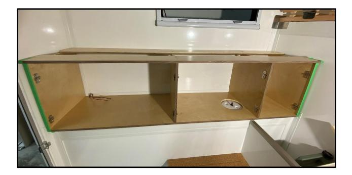
An expanded view of the different components is shown below. The upright pieces (gables) can be glued and screwed through the top and bottom pieces.
