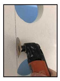
8. Use knife to cut through foam and remove panel.
