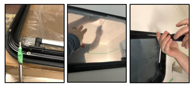
12. Install clips facing upwards. The rail on back of blinds fits into the clips.
