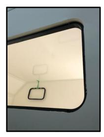
10. Remove all dust and dirt from surfaces using brush and rag with denatured alcohol (other cleaners can damage fiberglass). If dust gets on window seal it can lead to potential leaks in the future.
