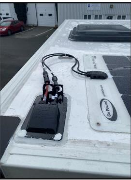
The solar wires will come down through the roof like in the photo below. We built a small wood box above the cabinet that can slide flush to the wall to hide the wires.
