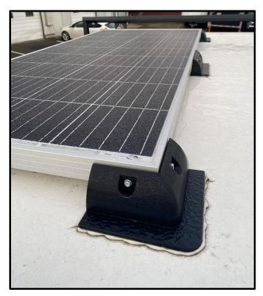
The plastic drill free mounting brackets can be purchased from amazon. Make sure to lightly sand the mounting bracket and the area on the roof panel that the mounting bracket will sit. Before gluing, clean all surfaces with solvable methyl hydrate and a clean rag.
