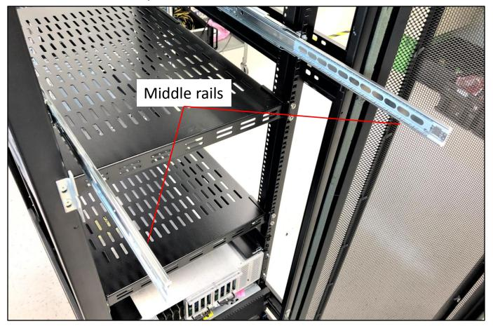
After extending the Middle rails, you can now mount the chassis enclosure. Align the back-end Inner rails from the chassis to the Middle rails.
