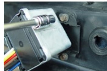
Photo 25. This photo is an inside the dash shot of installing a 1969 and later Delay Switch.
