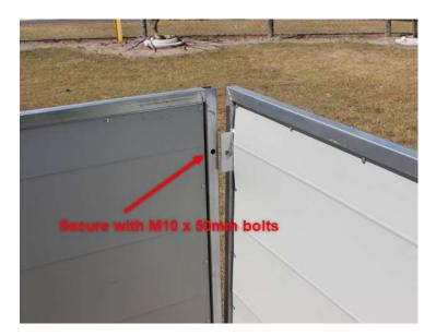
**Step 4.**Measure the diagonal corners of the unit, adjusting until the measurements are the same and the frames are square. Then tighten all bolts firmly.
