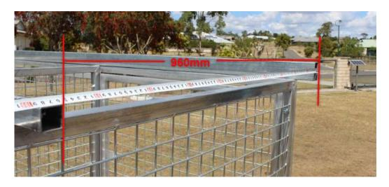
The second middle roof bearer MUST go in front (towards the front of the kennel) of the original middle roof bearer that was measured back 960mm.
