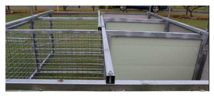
Recheck diagonal measurements are still equal. If they are not, adjust until unit is square. Then tighten all bolts firmly – unit must be square and all bolts must be tightened before the next step.
