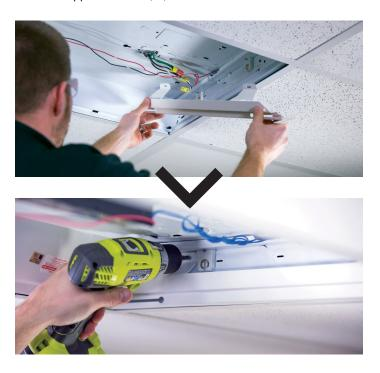
**3. Optional:** Install side plates (x2). This is dependent on whether or not there are gaps between the fixture and the existing ceiling grid.
