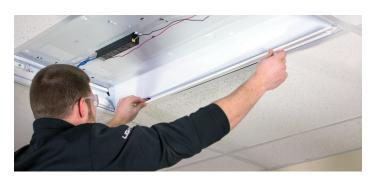
**4.** Insert the doorframe of the retrofit into the keyholes of the support brackets and slide the unit into place.
