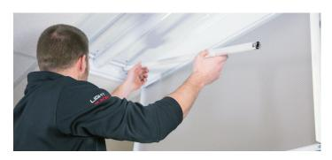
**2.** Install support brackets (x2) and secure with tek screws.
