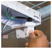
**3.** Break apart the 1-piece mounting bracket kit into 3 individual pieces. Install a small bracket to each end of the fixture and the large bracket at the center of fixture (for 8' fixtures only) by bending them over the fixture to fit the exact width and fastening them to the fixture with the provided tek screws.
