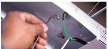
**5.** Make electrical connections for input power (via the included Power Quick Disconnect) and fixture ground. 0-10V connections optional. **For 8' kits only:** connect the LED module wiring between the 2 strip pans via the pre-wired linking connector.
