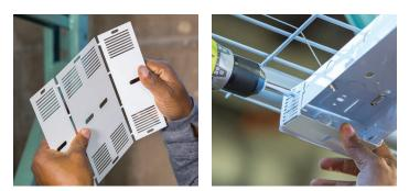
**4.** Fasten the safety cables (x2) from the retrofit pan(s) to the fixture housing using existing lances/holes of the fixture.
