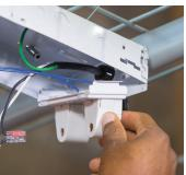
**3.** Break apart the 1-piece mounting bracket kit into 2 individual pieces. Install the brackets to each end of the fixture by bending them over the fixture to fit the exact width and fastening them to the fixture with the provided tek screws.
