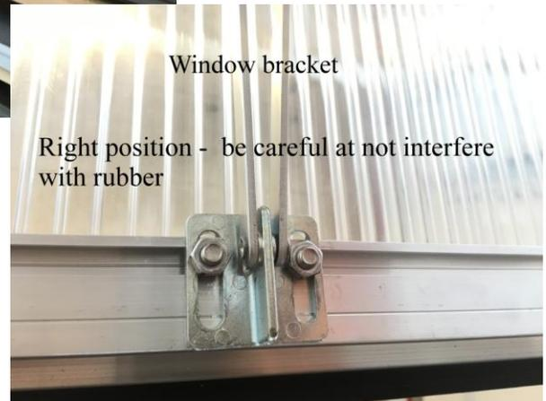
In the correct position, the opener is sitting parallel to the window, which means that it will not demand a lot of pressure from the cylinder when the opening starts. Before fitting a new cylinder to the openers, you must check that the window can open freely right from the start. If not you must change the position of the aluminum profiles.
