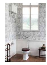
High-level pan with high level cistern and high-level angled flush pipe
