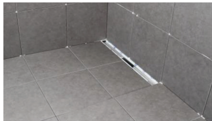
Apply grout between tiles.
