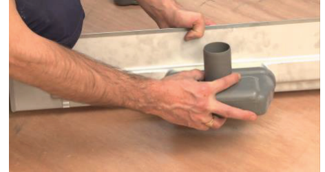
Place outlet onto the main drain body and clip into position.
