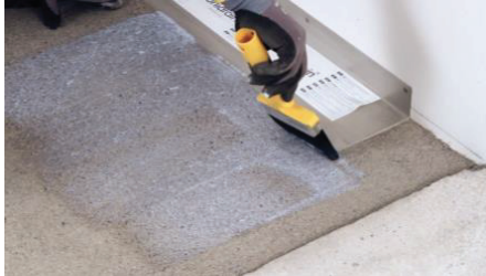
Apply Primer using brush or roller. Follow dilution ratios and zones below.
