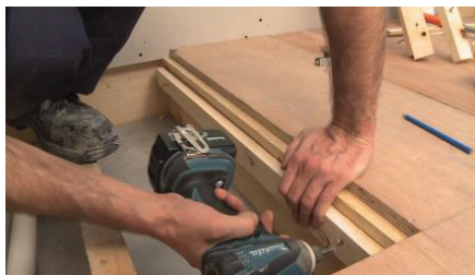
Install battens between the joists.
