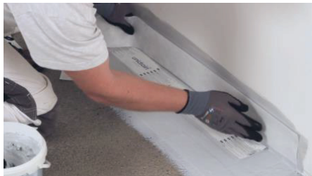
Apply VS30 using a brush or roller to all major joints. Place reinforcement tape into position.
