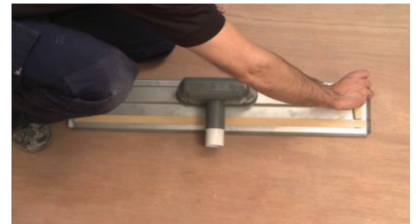
Place onto the bottom of the main drain body.
