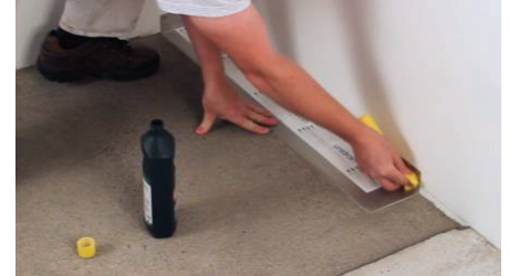
Degrease the drain using a degreasing agent.
