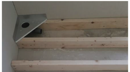
Screw drain to wall using screws supplied
