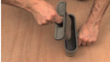
Remove the trap from the top of the outlet.
