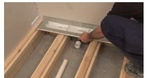
Screw drain to wall using screws supplied and connect pipework.
