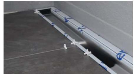
Ensure tiles come up to the frame but leaving a gap for grouting.
