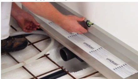
Place drain into position ensuring it is level.
