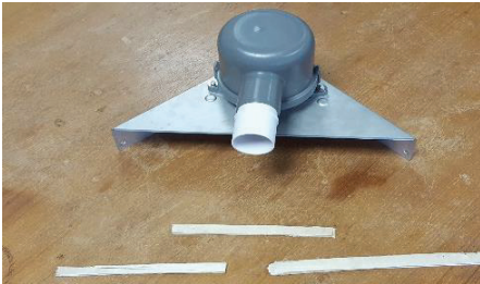
Cut three battens to size.
