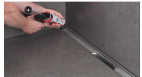
Seal all major joints with an anti fungal silicone.
