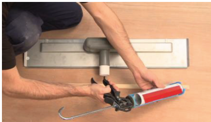
Apply glue to the battens.
