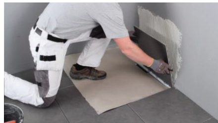
Tile the walls starting from the drain up making sure the tiles come down to the frame.
