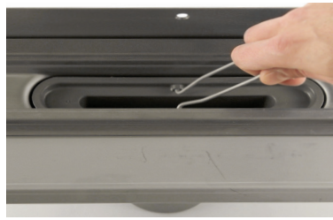
2. Remove the water trap
