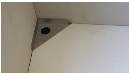
Screw the Unislope board into position using dry wall screws.
