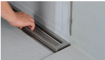
Place frame into position before you start tiling.
