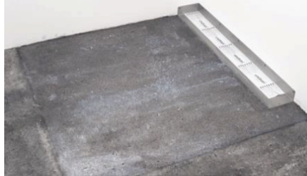
Allow approximately 30 minutes for Primer to dry. Ensure it is touch dry.
