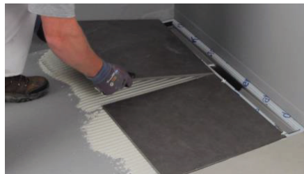
Tile to floor following standard tiling guidelines.
