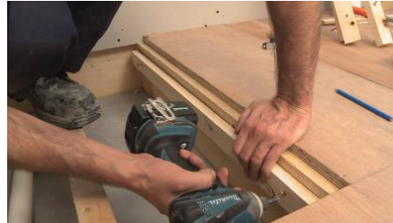
Install batons between the joist.
