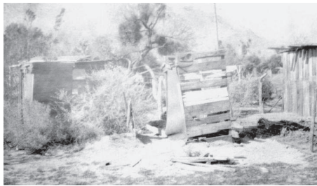
Debris and remains of abandoned building in Section 14 circa 1955.
