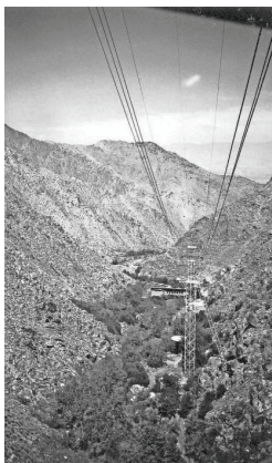
Palm Springs Aerial Tramway towers and view of the Valley Station.
