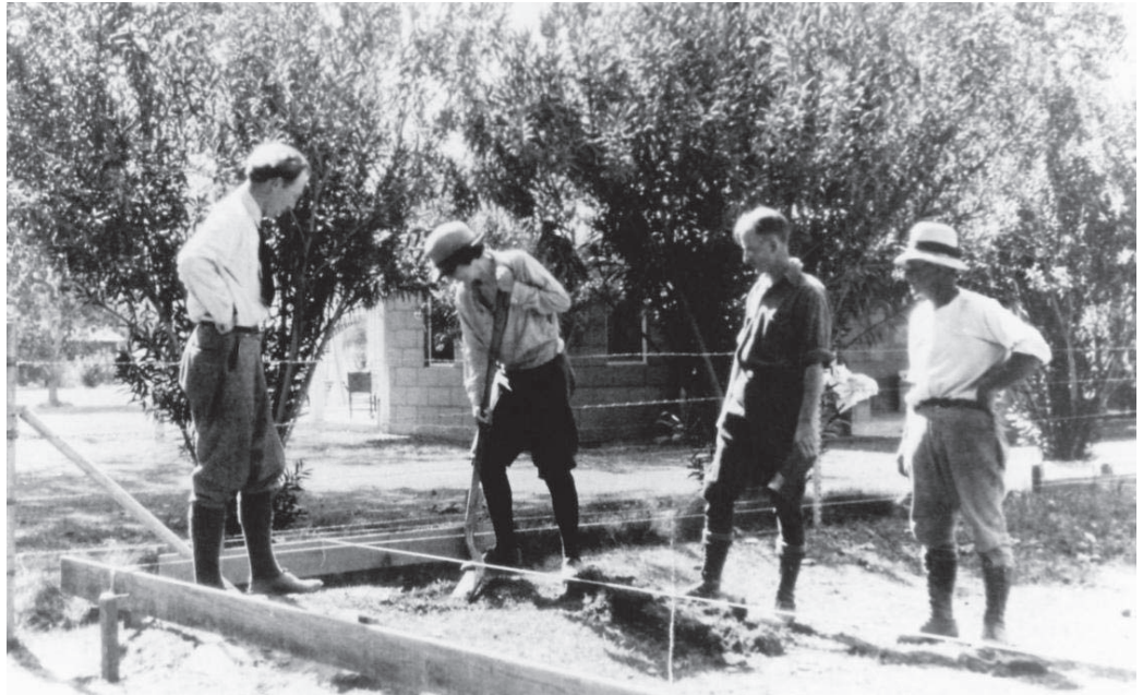
Architect Lloyd Wright, Pearl McCallum McManus, Austin McManus and contractor Quinn Spalding turn the first spadeful of dirt for the Oasis Hotel 121 South Palm Canyon Drive in 1924. PHOTO COURTESY OF THE PALM SPRINGS HISTORICAL SOCIETY
