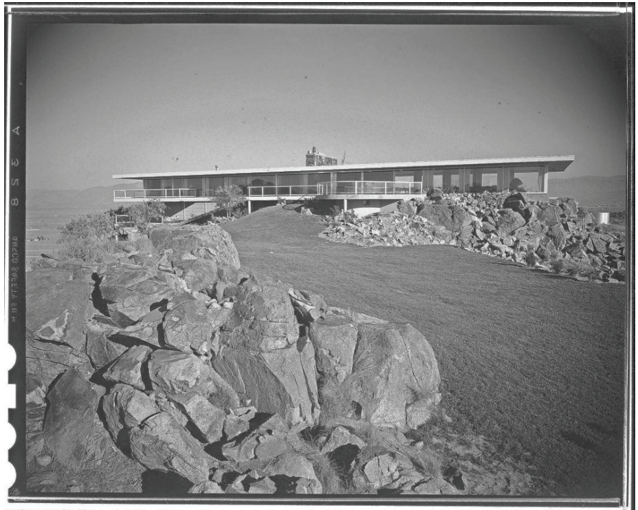
The recently demolished Hilltop House perched above Apple Valley as designed by Francisco Artigas and landscaped by Tommy Tomson. PROVIDED BY THE MAYNARD PARKER PHOTOGRAPHY COLLECTION AT THE HUNTINGTON LIBRARY
