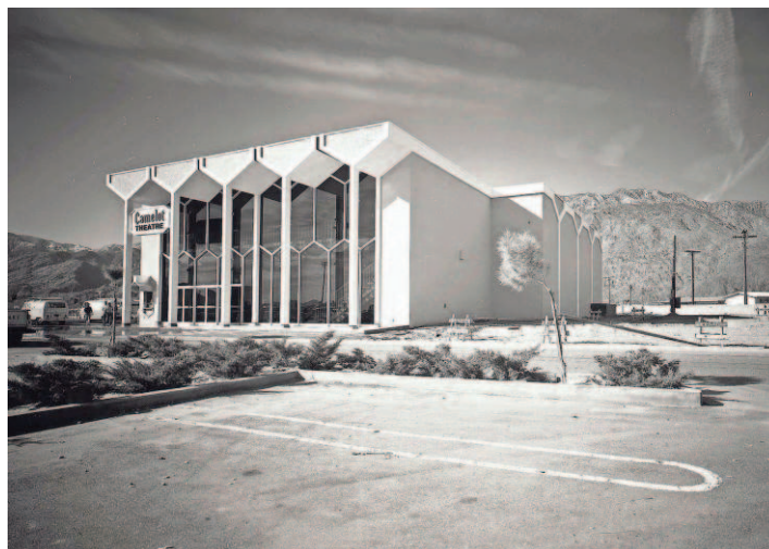
The Camelot Theatre, on Baristo near Farrell in Palm Springs, soon after completion of construction. COURTESY PALM SPRINGS HISTORICAL SOCIETY
