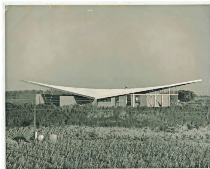
The Willcockson residence still stands, and its roof reaches to the heavens in seemingly silent prayer. COURTESY WALTER S. WHITE PAPERS AT UC SANTA BARBARA, ART, DESIGN AND ARCHITECTURE MUSEUM
