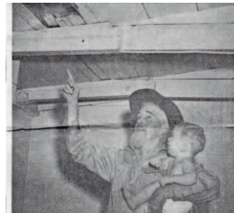
The box car schoolhouse pictured in its dilapidated state before demolition.
