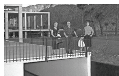
Underground parking for the golf course was a unique feature of the Eldorado Country Club clubhouse that was designed by Cody.
