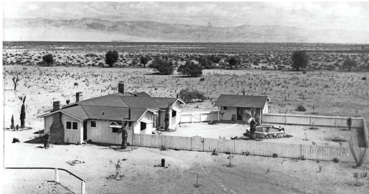
Deep Well Ranch in 1925 consisted of a few buildings and the eponymous well.
