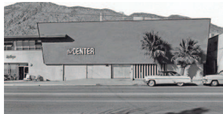
The Town and Country Center had a dramatic east façade.
