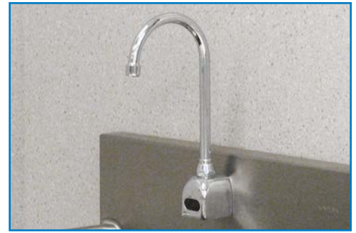
OA-204 - HANDS FREE MIXING FAUCET Toggle a steady stream of water with this motion activated sensor.
