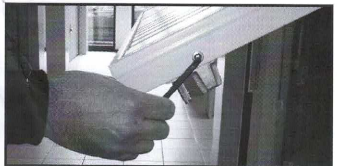
Locate latch spigot into relevant hole in boundary chassis from inside and then insert and tighten panel pivot bolts from outside.
