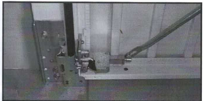
Slide the locking bar onto the lug on the back face of the latch. (Once located it should slide freely)
