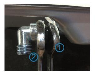
B: Look tightly a replaceable gas-type fitting onto the main gas tube.
