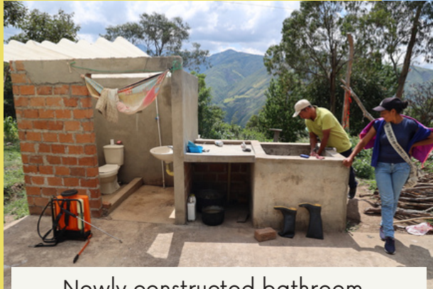
Newly constructed bathroom.
