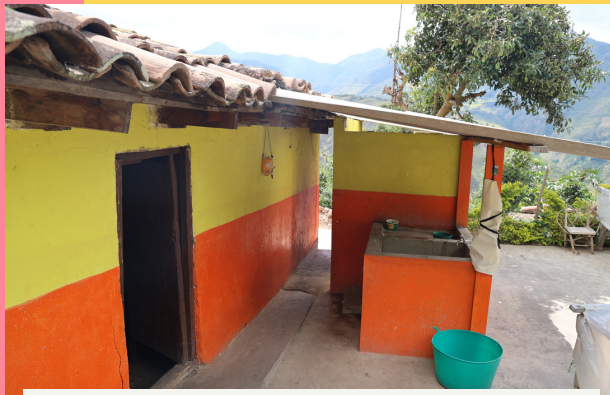
Newly constructed bathroom.
