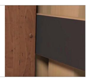
If a roof trim is used to finish your installation, leave a 5mm gap between the top of the cladding planks and the trim.
