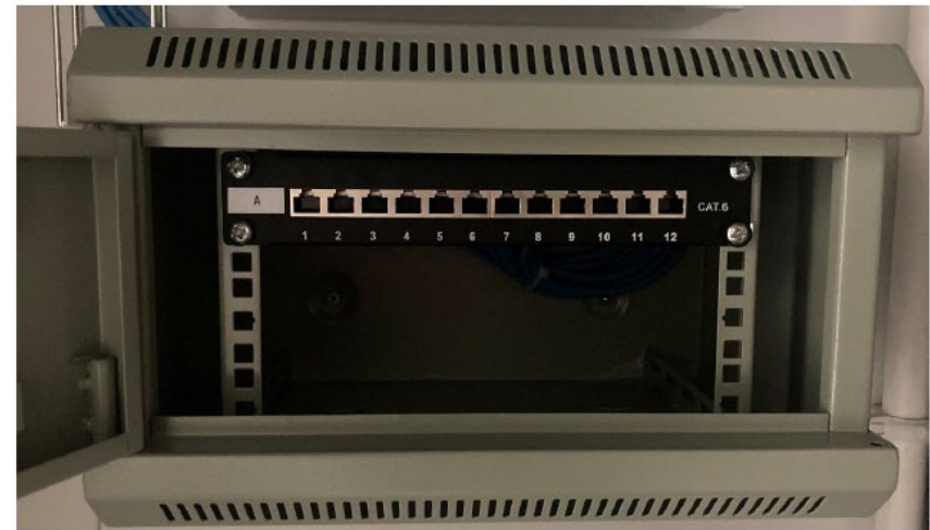
Figure 8 Patch-panel box
