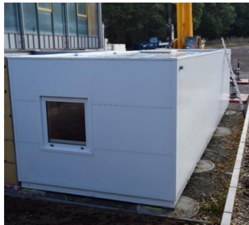
Figure 7 Block foundation
