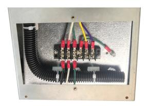
**D.** When using the supplied plug-in cord, match the cord wiring color to the same color wires on the wiring terminal block.
