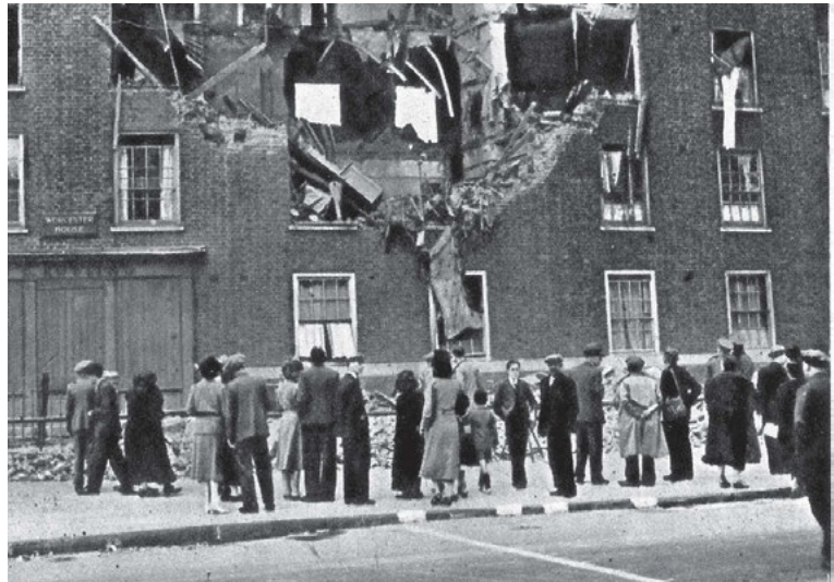
A block of flats in Kennington Road, Lambeth 8 September 1940 from Front Line.
