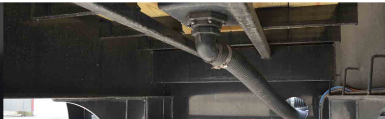
All Plumbing Under the Deck
