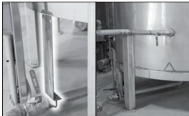
Fig 8 - Bracket to support piping from bottom coupler
