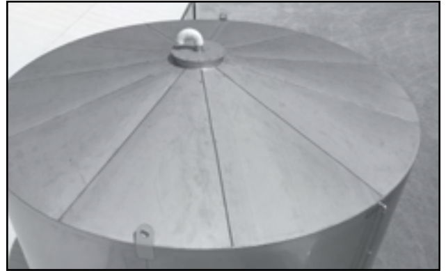
Fig 9 - Top of tank
