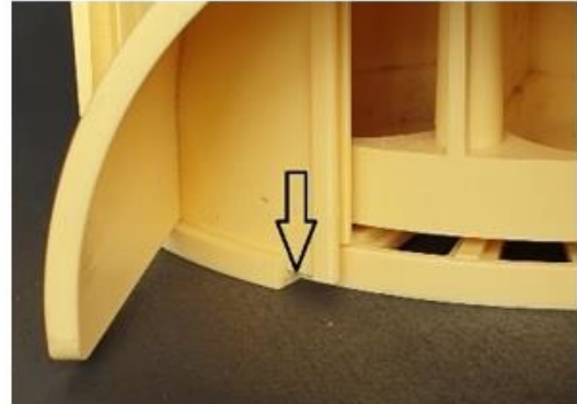
Top inserted fully into groove of bottom plate.
