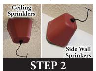
Always check for fire sprinkler's installed in a building. Keep heat level at fire sprinkler head a minimum of 30F below the trigger temperature
