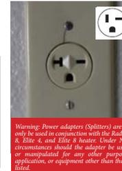
Each heating element draws 8 amps or 960 watts. Two (2) heating elements can be plugged into a 20 amp circuit or One (1) heating element per 15 amp 110 volt circuit.
