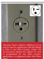
Each heating element draws 8 amps or 960 watts. Two (2) heating elements can be plugged into a 20 amp circuit or One (1) heating element per 15 amp 110 volt circuit.
