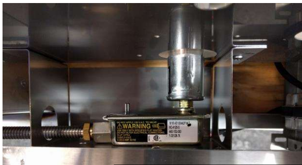
Correct installation The gas valve orifice is completely inserted inside the venturi
