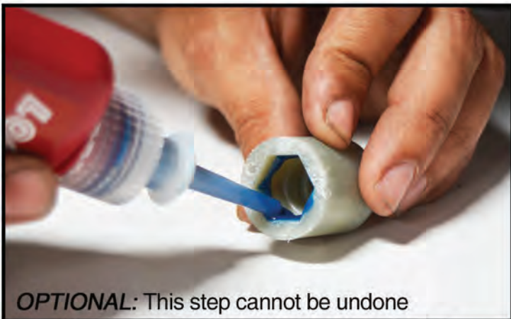
21 Use a sealant around the inside of the plastic coupling for a tight fit
