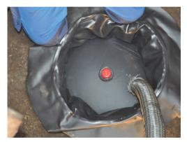
10. Pull the cylindrical part of the manhole neck to the top and through the manhole.
