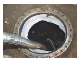
8. Glue the sealing strip made of foam rubber into the manhole neck.
