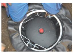
11. Using the fastening ring, brace the manhole neck of the inner lining against the foam rubber glued into the dome neck.
