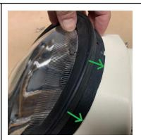
b) Align the trim rim screw hole with the top hole and put back the screw in place without tightening the screw too much to avoid cracking the plastic parts.
