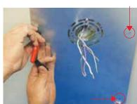
10. Attach the LED light panel to the mounting plate by inserting the hooks on the mounting plate into the slots on the back of the light panel. Once the hooks are inserted. slide the LED light panel until it is securely in place.
