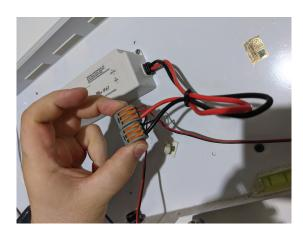
7. Connect the AC input wires on the driver to the AC power cable that supplies power to the mirror. Connect the white(neutral wire) from the AC power cable to the blue wire on the driver and connect the black(line wire) from the AC power cable to the brown wire on the driver. (These connections should be made using the existing Wago connectors)
