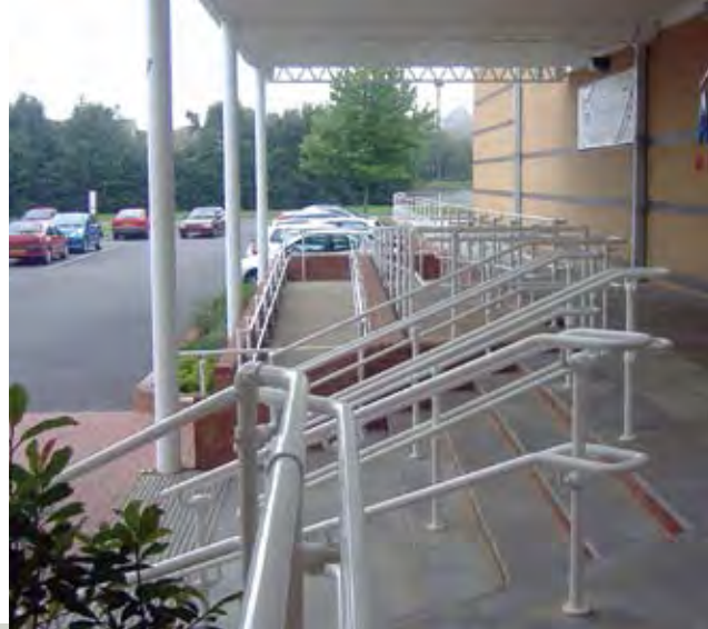
Right: ADA Compliant Railing for Public Access
