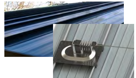
Standing Seam Roof
